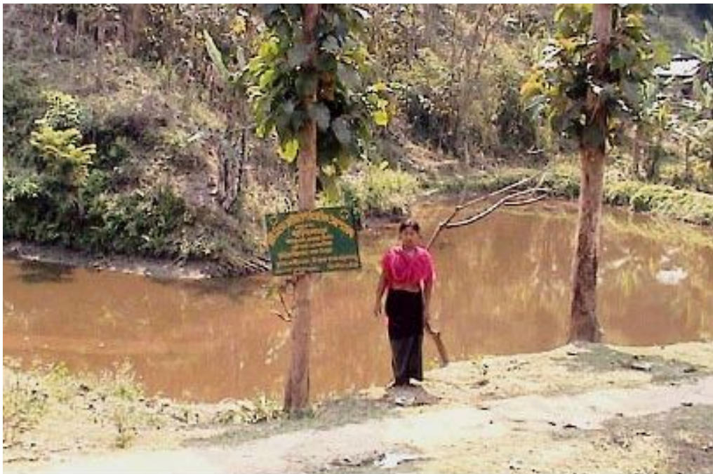
Water harvesting structure of Smt Sakhibala Jamatia
